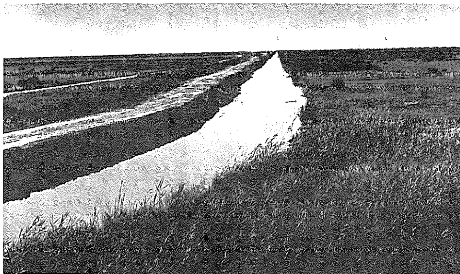
NAD-I-ALI AREA drain and wasteway illustrates the need of such facilities to prevent waterlogging of farm lands.
