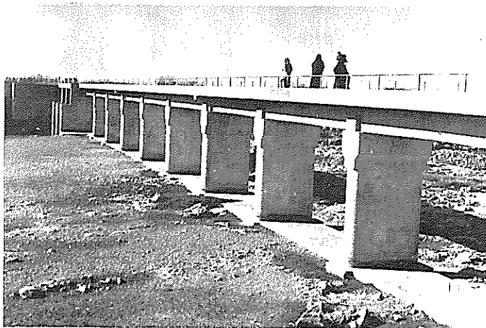
ARGHANDAB RIVER water is diverted to the Zahir Shah Canal at this bridge.
