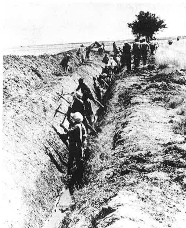
Figure 5-13 Excavating a Drainage Channel
