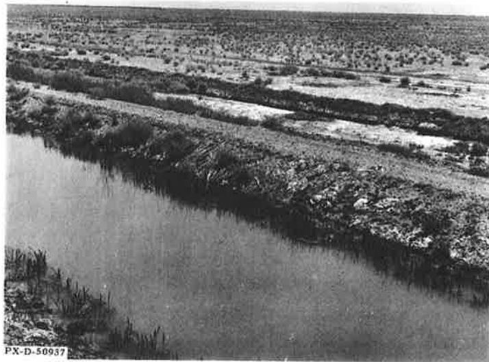
Figure 15. --A typical shallow drain associated with saline-alkali soils shows that the area needs better drainage to relieve water table.
