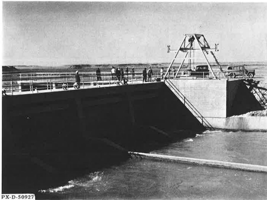
Figure 4. --This diversion dam takes water from the Helmand River and directs it into the head of one of the large canals. It replaces many hand-built rock and brush dams which had to be rebuilt each year.
