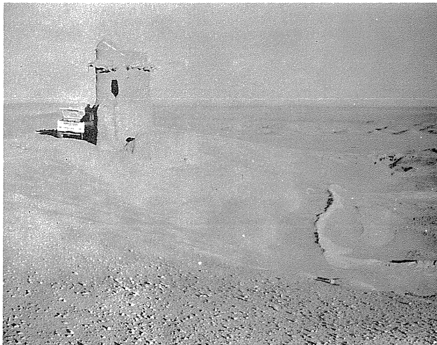
Nur Mohammad Band with tower. Note piles of earth in drainage area in background. A much larger drainage area is to the right.
