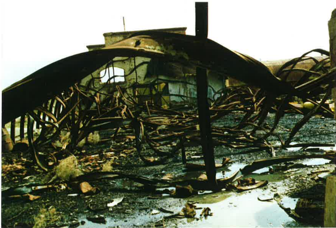
29. Spare parts warehouse at Chan-i-Anjir equipment yard, 18 March 97
