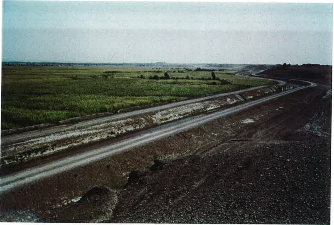
39. The S-10.7 lateral under construction, 1972
