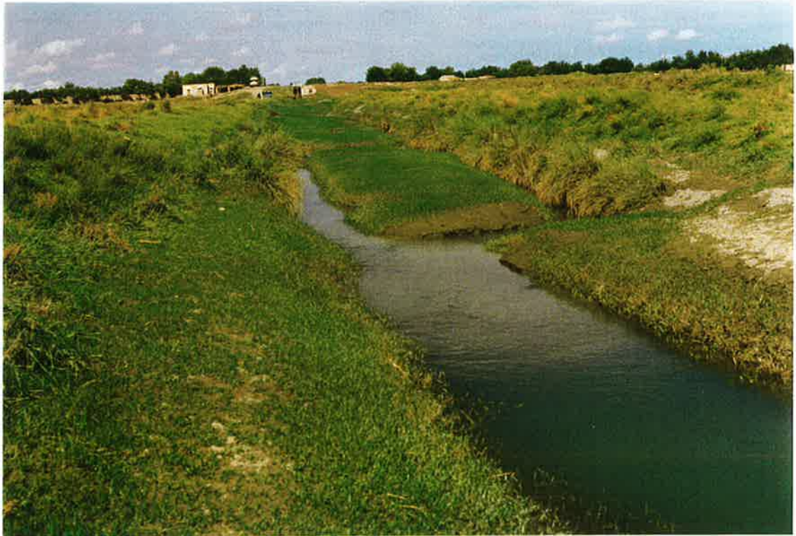
44. Silted lower Shamslan Canal, 17 Oct 97
