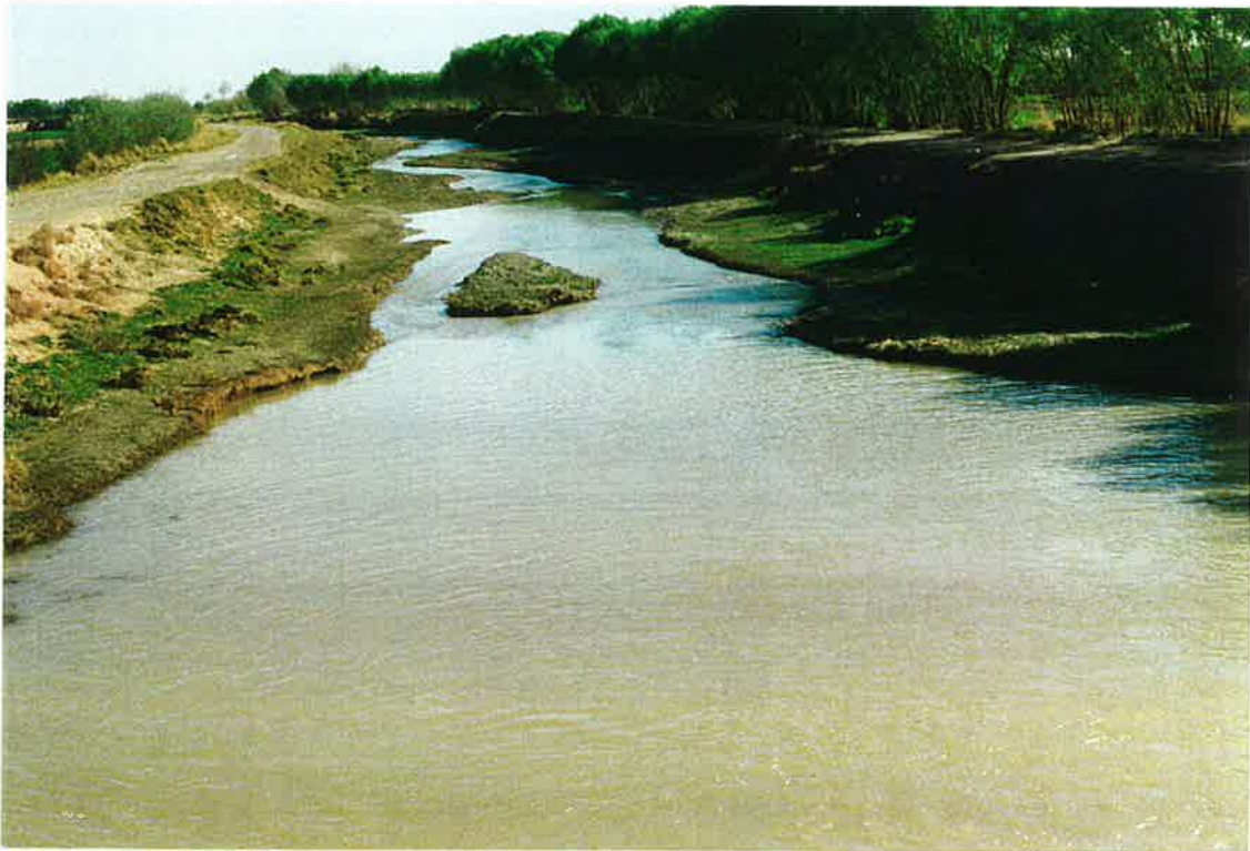
34. Shamalan canal looking south at the S-10,7 lateral intake. Note silting. 21 March 97
