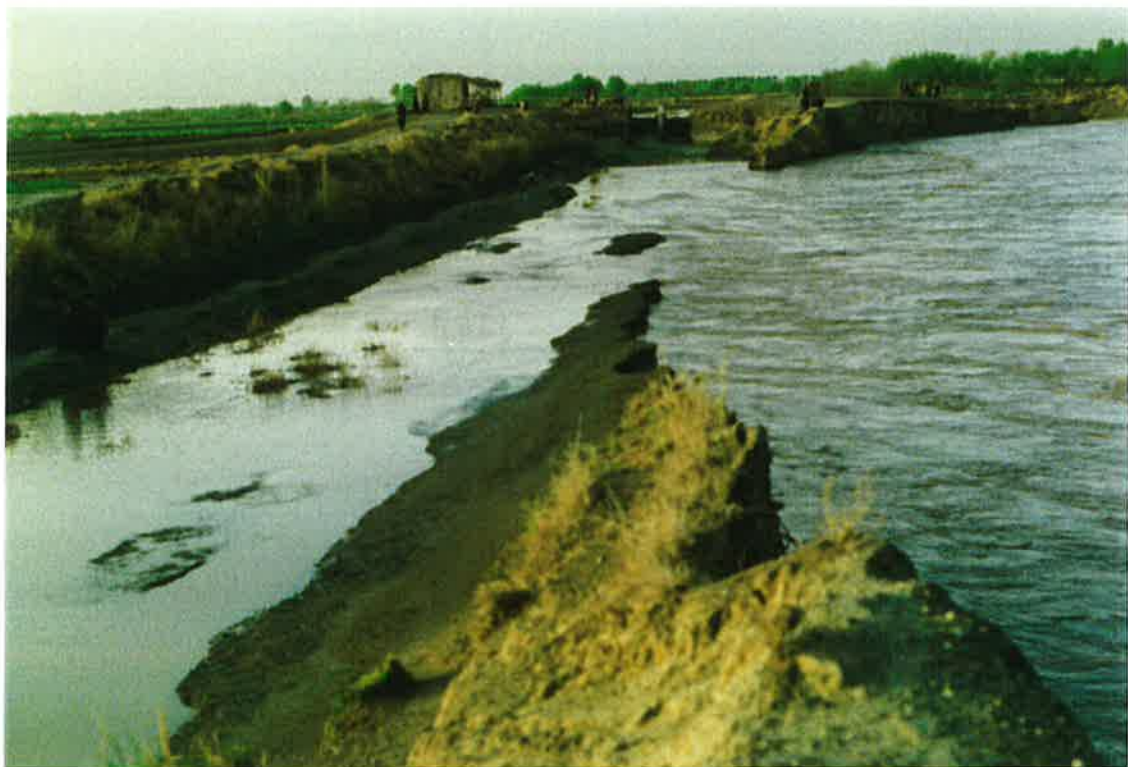
36. Helmand River (on right) at wash out of Shamalan canal just below Waste way #1, 17 March 97
