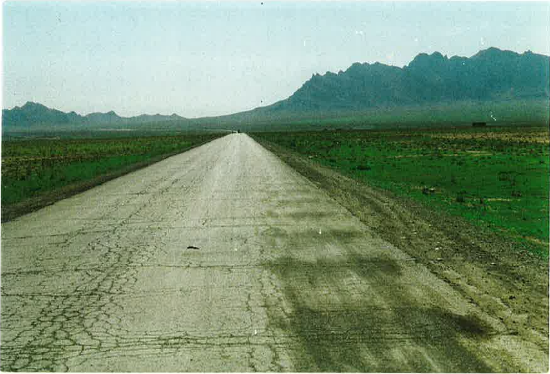
1. Chaman to Kandahar highway 26 March 97
