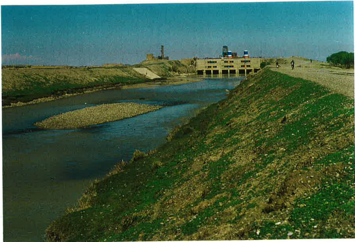
76. Girishk power plant with silt on Boghra canal, downstream side. 20 March 97
