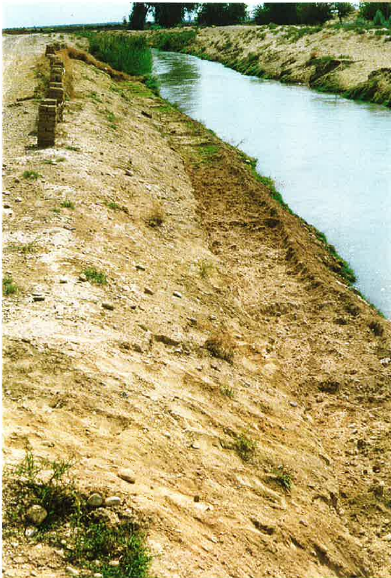
108. Excavated vegetable plot on silt embankment on Boghra canal near Marja. 18 Oct 97
