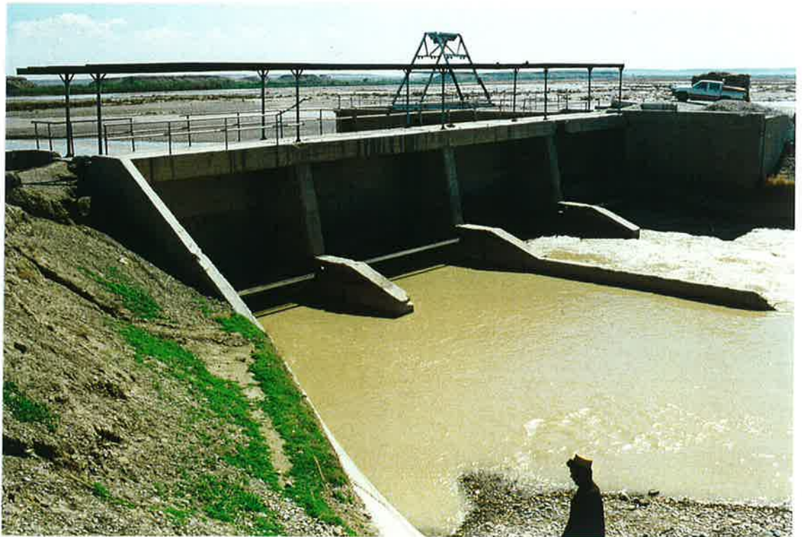
57. Baghra Canal intake structure on Helmand River with 2 gates open. 20 March 97
