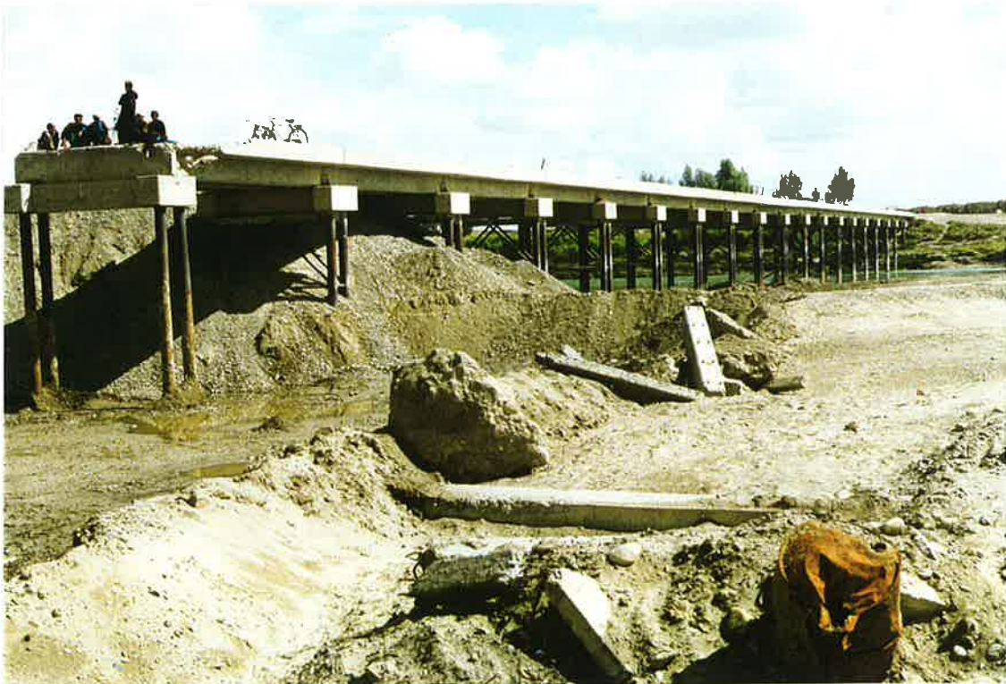
46. Darwishan Bridge looking east. Original structure intact. 17 Oct 97
