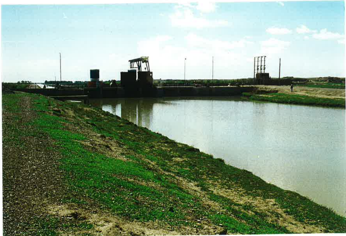
75. Girishk power plant on Boghra canal, up stream side. 20 March 97
