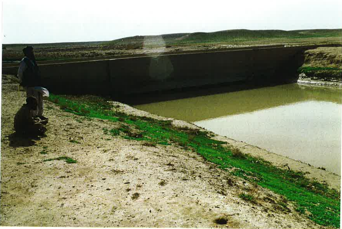
94. Wash crossing near Marja. Note silt embankments at water edge. 22 March 97
