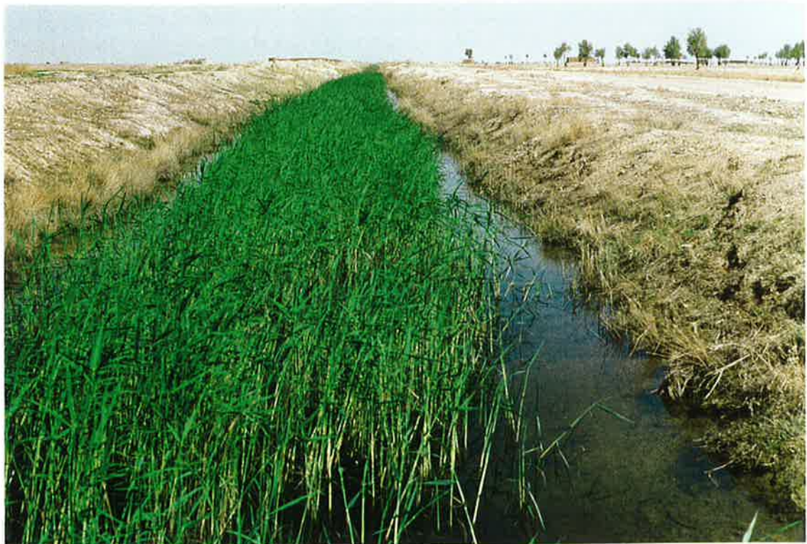
112. Un-maintained main drain near Marja. 22 March 97
