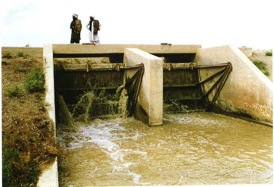
100. Waste way gates off Baghra canal near Marja, See # 99 above. 18 Oct 97
