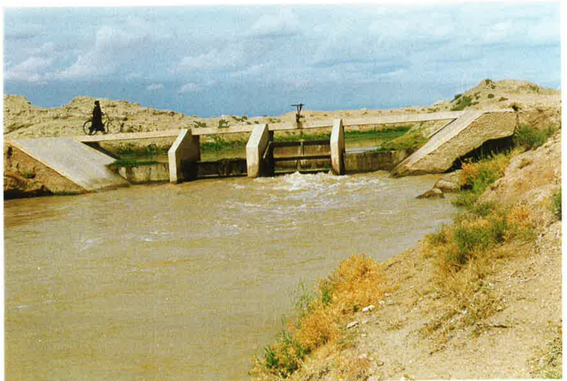
103. Damaged control structure on Boghra Canal near Marja. One gate functions. Note washed out wings. 18 Oct 97.
