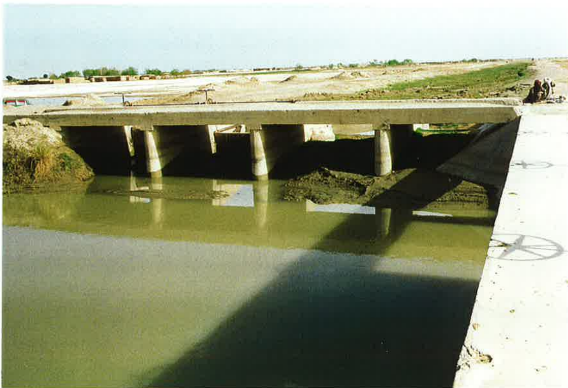
96. Silted waste way gates near Marja. 22 March 97
