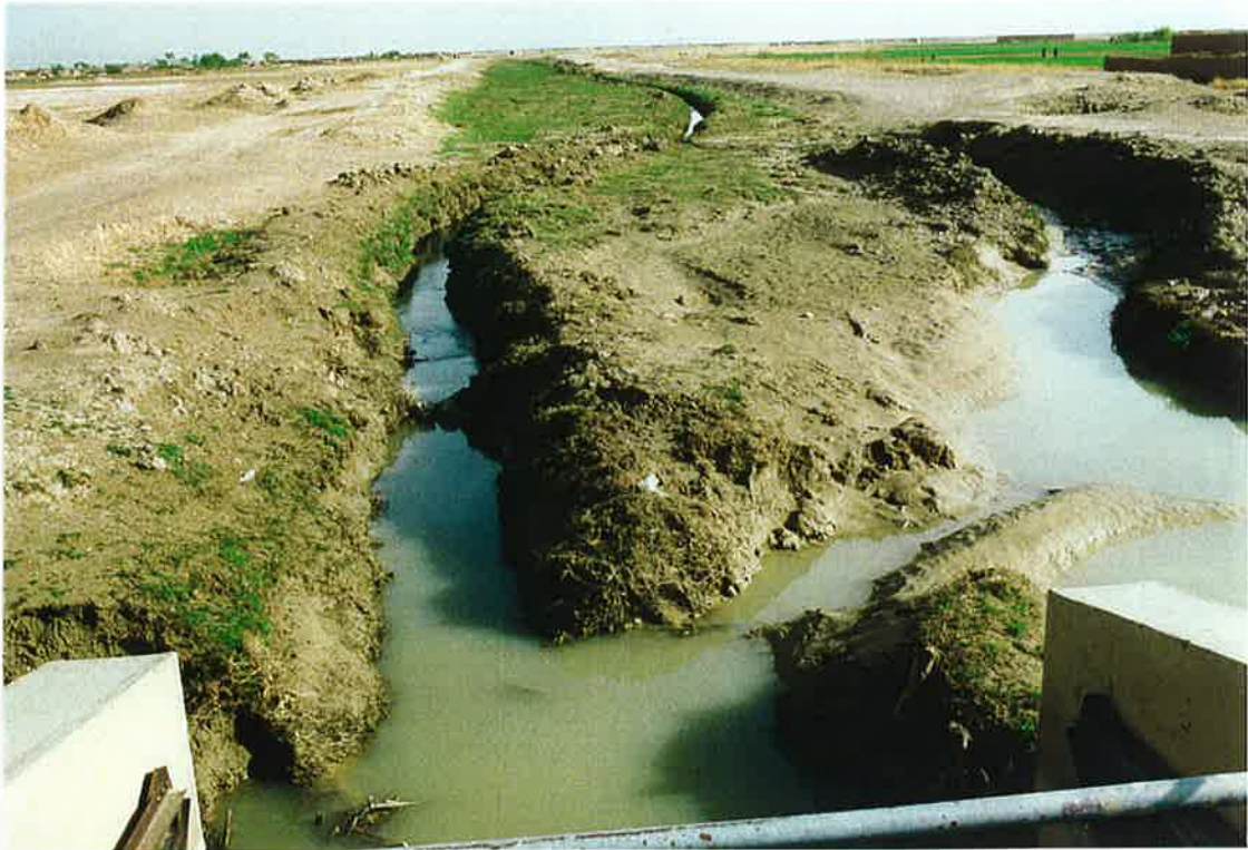
97. Farmer excavated irrigation ditches in silted bed of a wasteway near Marja. See # 95-96 above. 22 March 97
