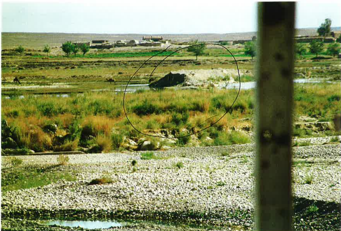
64. Close up of old failed MKA river diversion dike on Helmand River. 20 Oct 97
