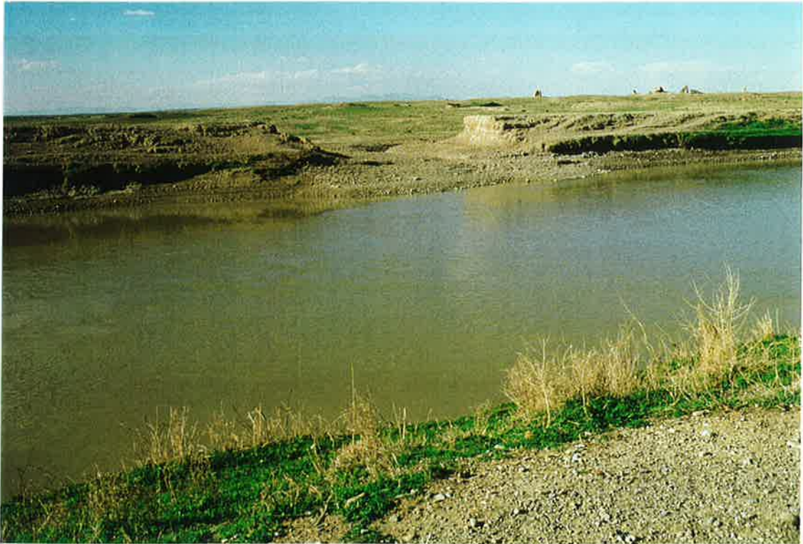
77. Excavated/breached Boghra canal embankment south of Girishk. 20 March 97
