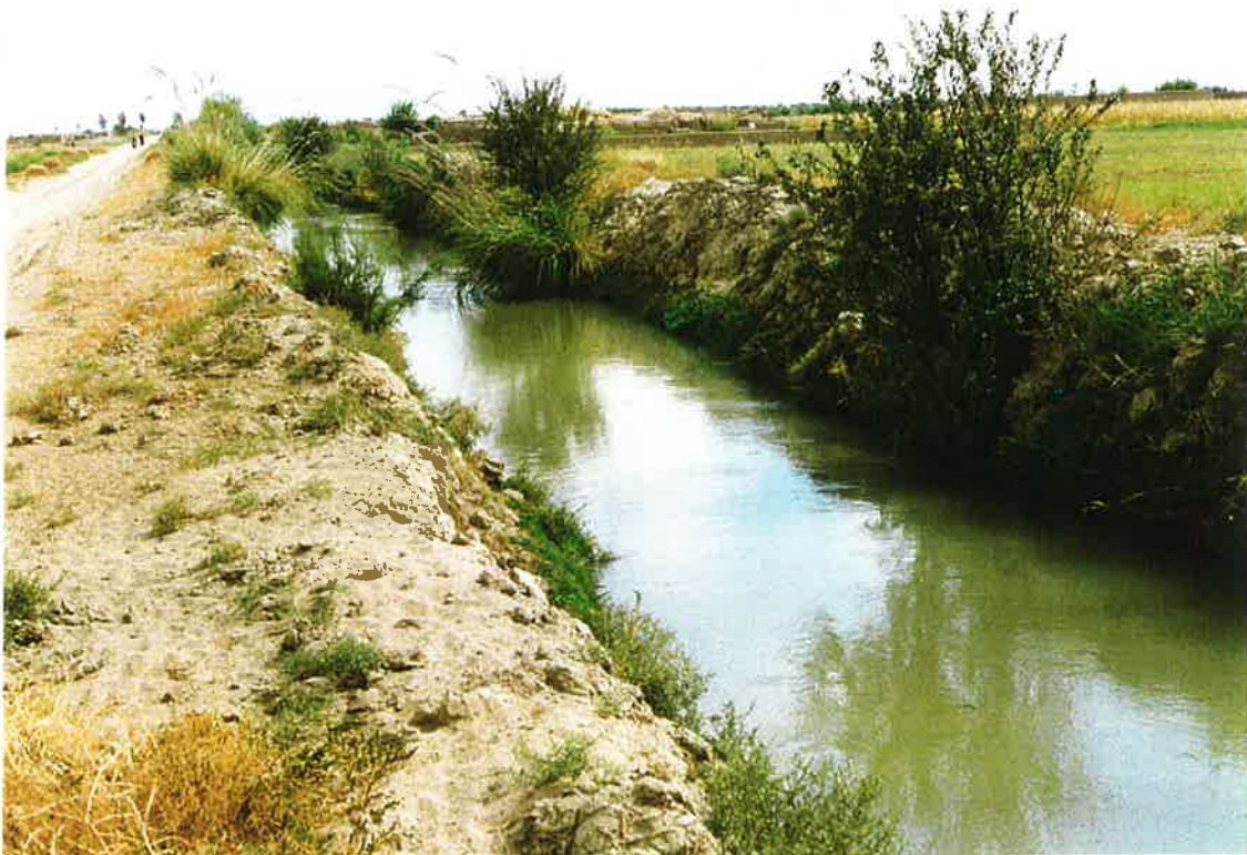
110. Central Marja channel cleaned by local water users organization. It needs more of the growth removed. 18 Oct 97
