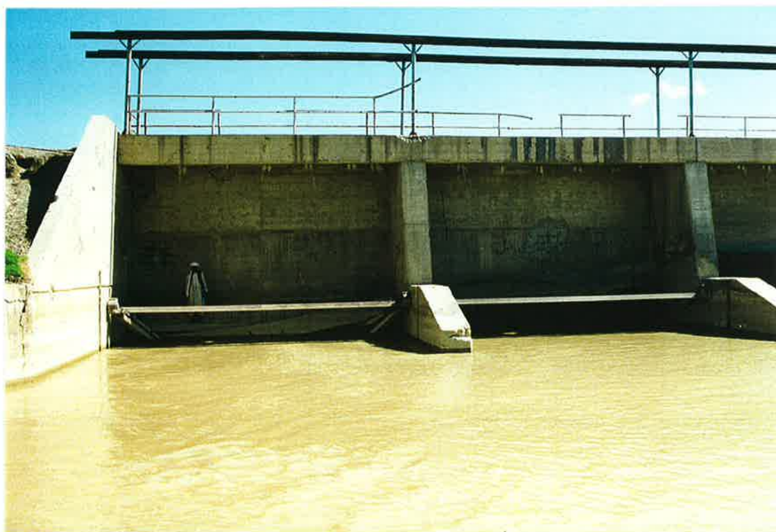
62. Two gates of Boghra Canal intake structure. 20 March 97
