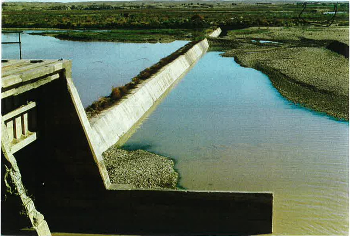
63. Old failed MKA river diversion dike (ca. 1947) on Helmand River From Boghra canal diversion structure at intake. Dike in upper right corner. 20 Oct 97
