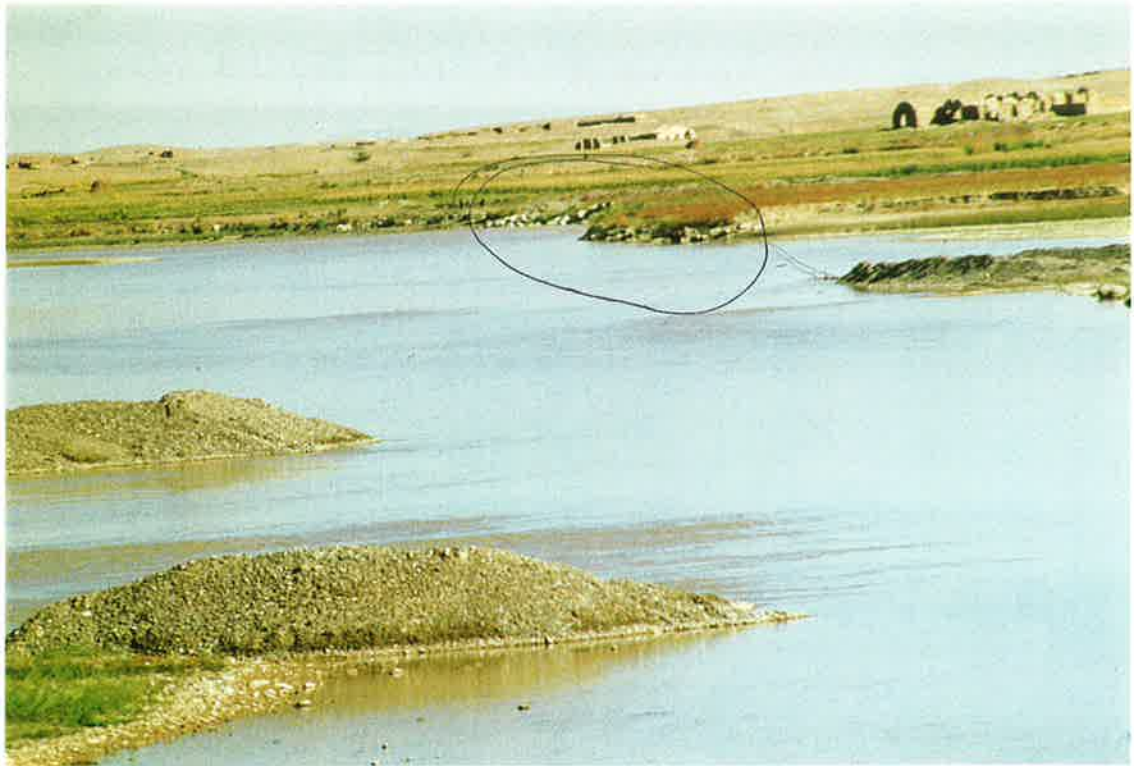
71. Close up looking north up Helmand River channel at location of old failed MKA upper river diversion dike from Boghra intake. Note large block base of old dike. 20 Oct 97
